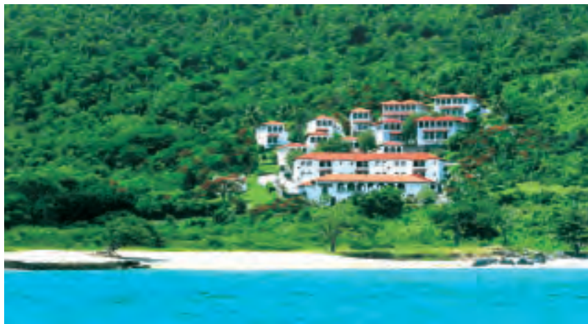
Above: The existing villas on the 30-acre site of the spectacularly positioned Mount Cinnamon resort
